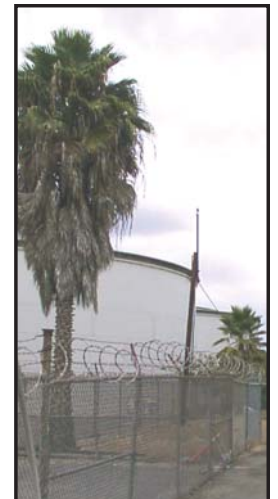
Each of the two water storage facilities is surrounded by razor wire topped fencing. Sensors alert the monitoring system to turn cameras to the location of any disturbances.
